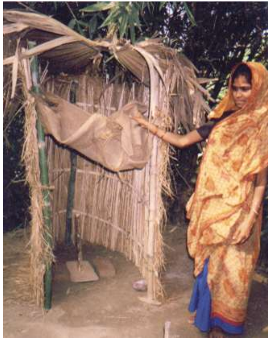
Simple pit latrine with wooden cover (Suzanne Hanchett photo, copyright PAC)
